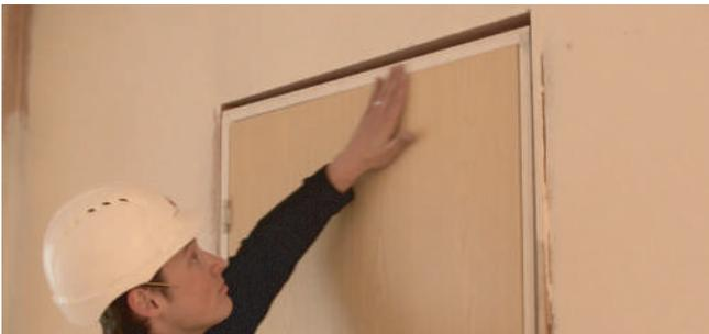
**7** Swing the 'Dummy' doors provided by removing the screws and cams from each of the female keeps, and slide it on to the male hinges on the frame. Check the head of the frame is square, and adjust where necessary by packing the jambs. (Note: Doors are susceptible to swelling, and some slight sizing may be necessary initially).
