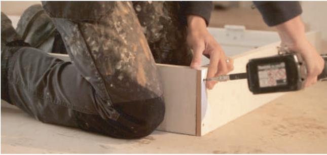
**5** Assemble the lining on a level surface - bearing in mind the handing of the door. Pre-drill pilot holes and screw the heads to the jambs with maximum 4x40mm long screws. Care should be taken to ensure that components are aligned correctly, and that the ironmongery is positioned as required.
