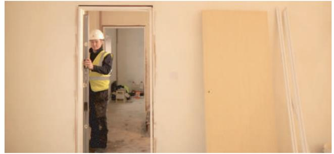
**6** Position the assembled frame into the opening. Ensure that the hinge jamb is plumb. Temporarily fix with two 70 mm long steel screws (minimum) ensuring the screw penetrates the wall by a minimum of 45mm.
