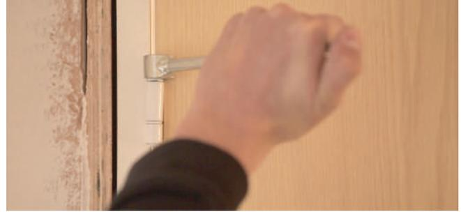
**8** Further adjustment can be made using the cranking tool provided. Apply slight pressure to the tops and bottoms of each hinge knuckle, to ease the door leaf towards or away from the latched jamb. A clear and consistent gap should be achieved all around the door.
